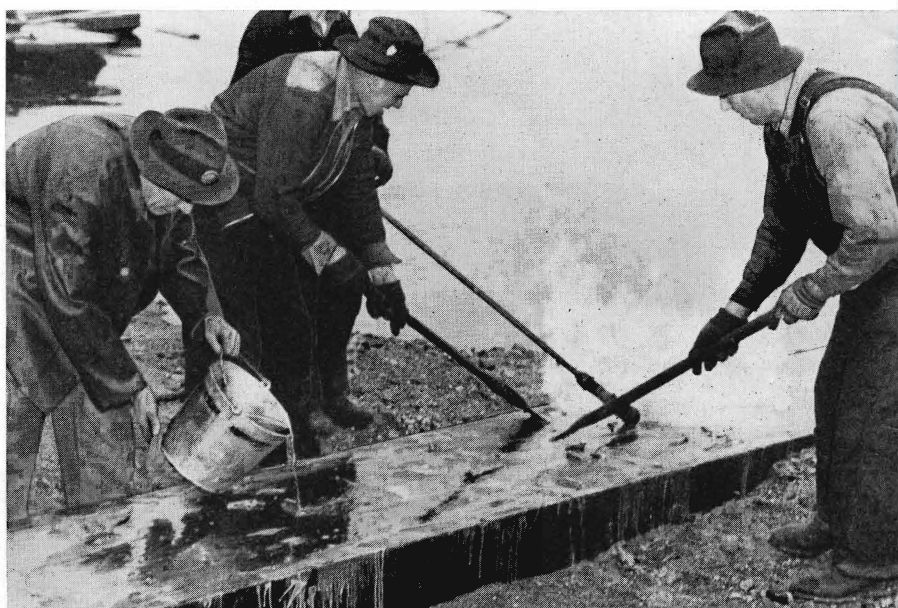
The melted base coat is applied while hot to the surface of the groundways. Successive layers of the hard, resistant grease are built up to support the weight of the ship.
