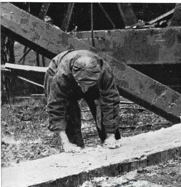
A softer, slippery grease, known as a slip coat, is applied to the base coat by hand or paddle.
