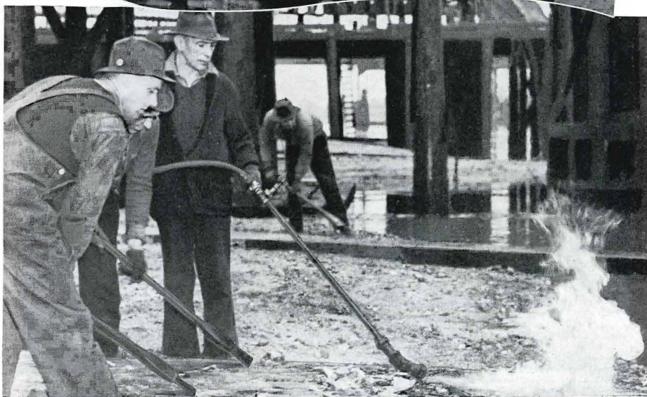
The ship safely launched, the surplus slip coat is salvaged. The ways are then prepared for the laying of the next keel.
