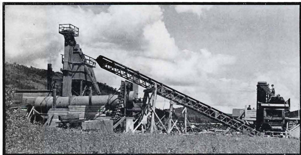
6 Towering above the countryside, the road-building equipment represents a big investment in machinery. At right is the mixing apparatus which blends materials for the road base. Left is the asphalt mixing plant where crushed rock, gravel and asphalt for the surface are combined.
