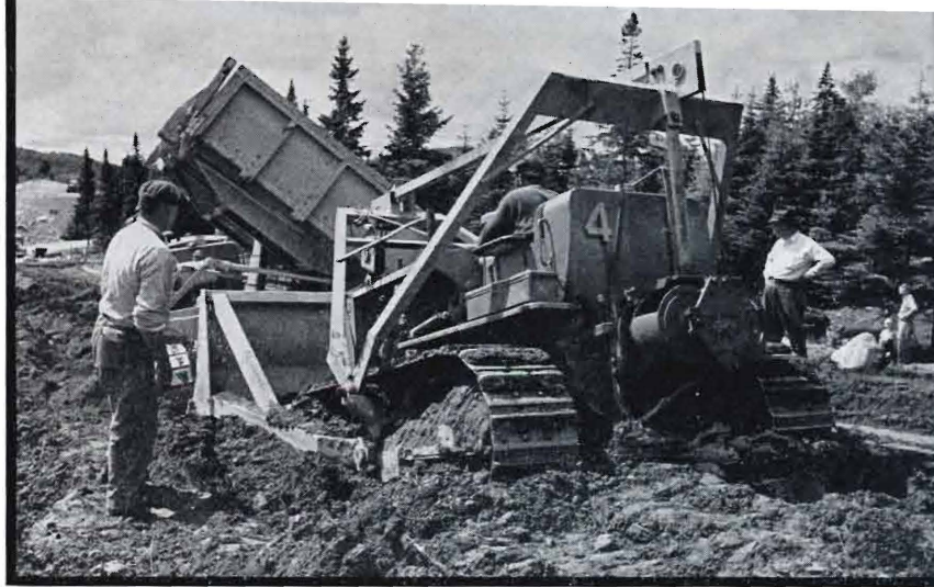
3 Powerful tractors pulling automatic unloading carts which carry 12 cubic yards of material at a time, bring in fill for the low spots—occasionally sink into the soft mud, have to be dug out.
