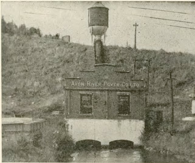
AVON NO. 1. This view shows the Power House in the foreground with the surge tank at the top of the hill.
