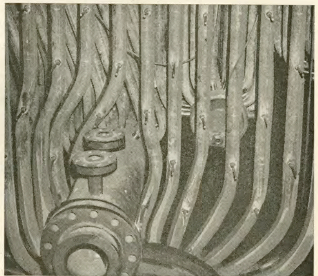
TEN MILES OF PIPE . . . enough to stretch from Halifax to Bedford . . . of which this is a section, is installed inside the huge boiler.
