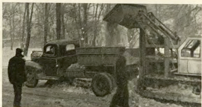
MECHANICAL ELBOW GREASE. This tractor-loader combination is used in order to speed up snow removal on tram-lines.
