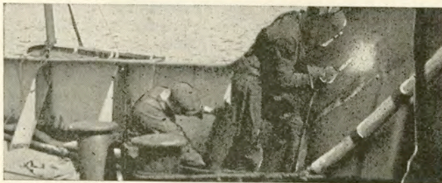
SPECIAL IRON CLAMPS designed by our Marine Department and adopted by the Admiralty, being welded to a ship's bulwark.
