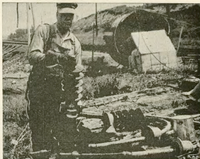
INSULATORS AND POTHEADS. Here a lineman is assembling the end fittings for a high voltage cable.
