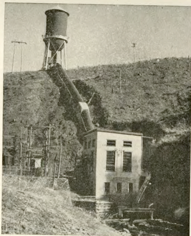
BLACK RIVER POWER HOUSE. A view showing the penstock and surge tank.
