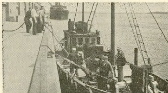
LOADING DEGAUSSING CABLE
