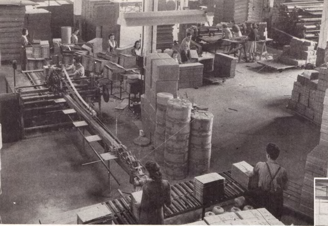
Automatic Taper is adaptable to all sizes of boxes, securing joints with heavy gummed cloth.
