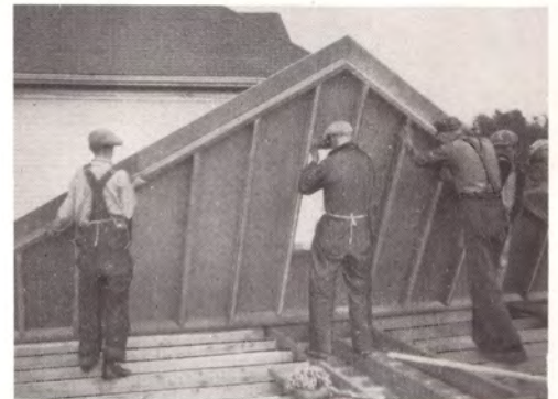
Gable end in one piece—slides into place.
