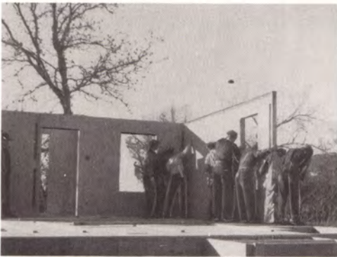
Finished wall panels fit.
