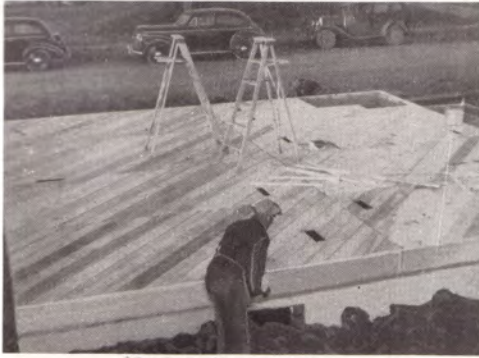
Floor sections in place.
