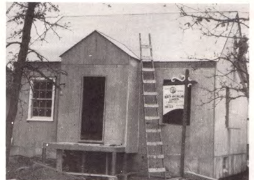
Ready for roof and exterior finish.
