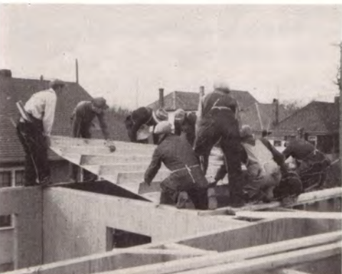
Ceiling sections built in large panels.
