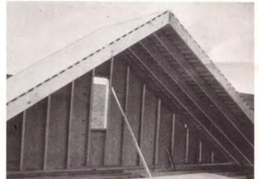
Roof panels take few minutes to erect.
