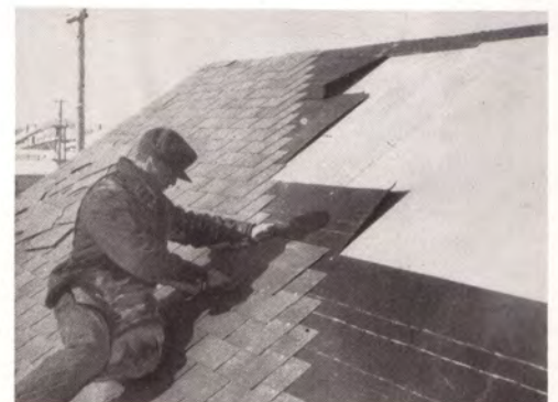
Shingles applied during afternoon.
