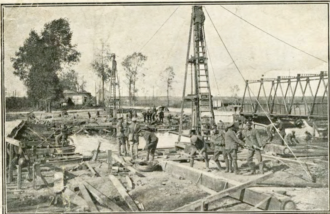
Canadian Engineers building an extra bridge across the Canal du Nord; the bridge on right was built by them in eight hours under heavy shell fire. Note pontoon bridge on left.
