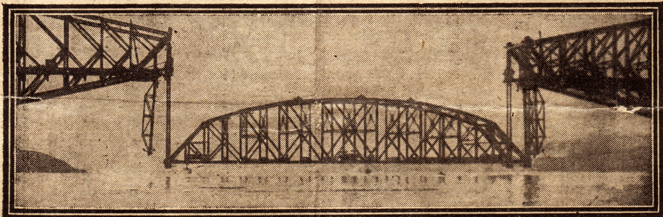
The five-thousand-ton centre span of the Quebec cantilever bridge—the largest of its kind in the world—ready to be hoisted into its final position. The picture shows the span just after it left the water on its journey of 150 feet upwards, which took four days.— Courtesy of the Dominion News Bureau.
