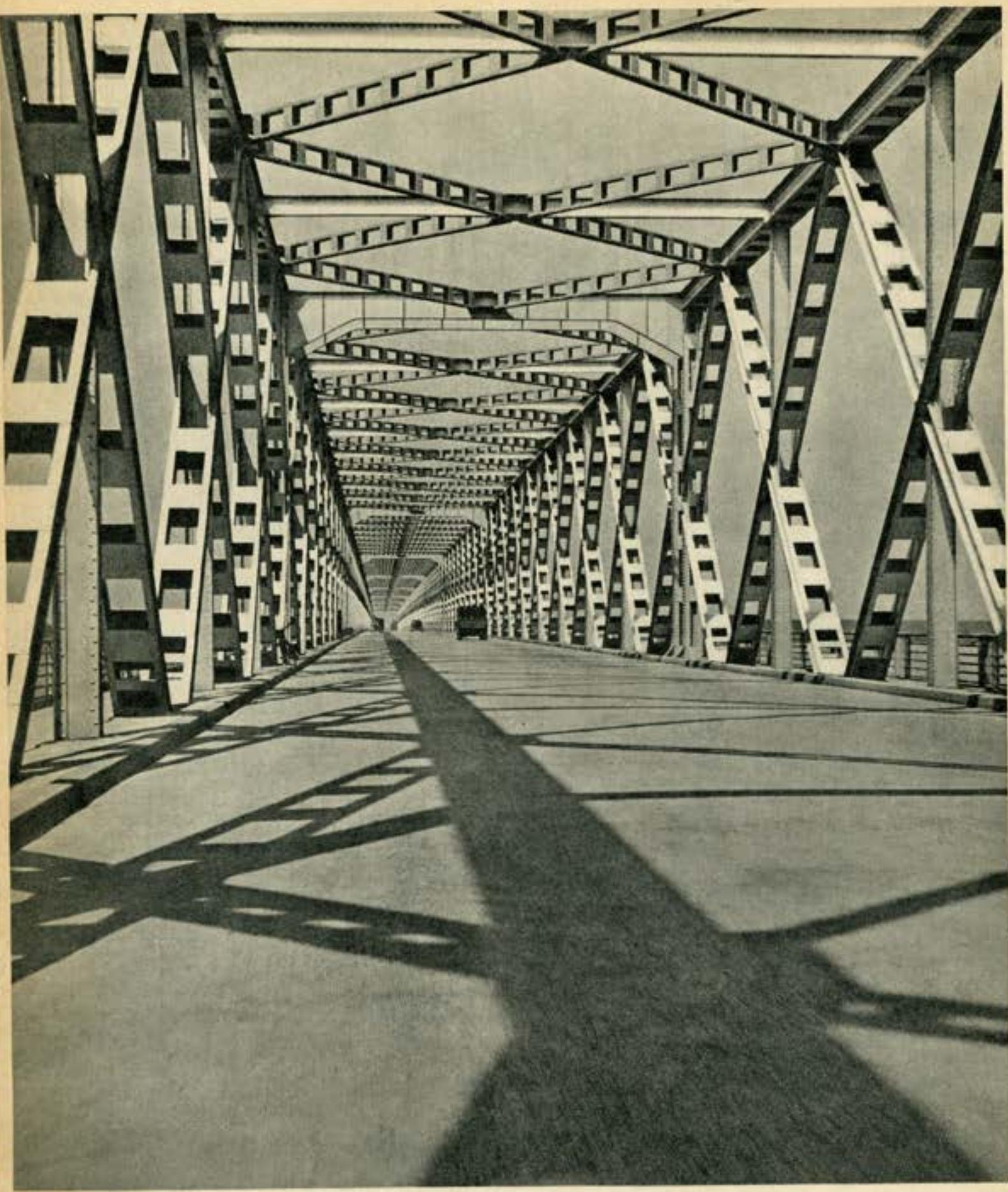
The Moerdijk bridges link the North of Holland to the South. This new traffic bridge, alongside the railway bridge, was erected in 1936, is more than 1000 yard long and 20 yard wide and has ten spans
