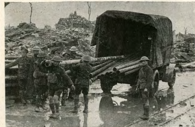
UNLOADING WATER PIPES.
