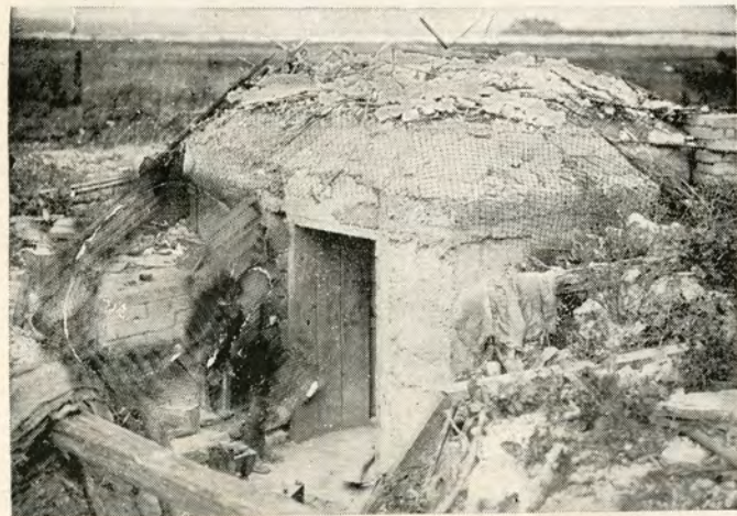
GERMAN DUG-OUT CONSTRUCTED WITH CONCRETE AND IRON GIRDERS, IN TRENCHES NEAR LENS CAPTURED BY THE CANADIANS.
