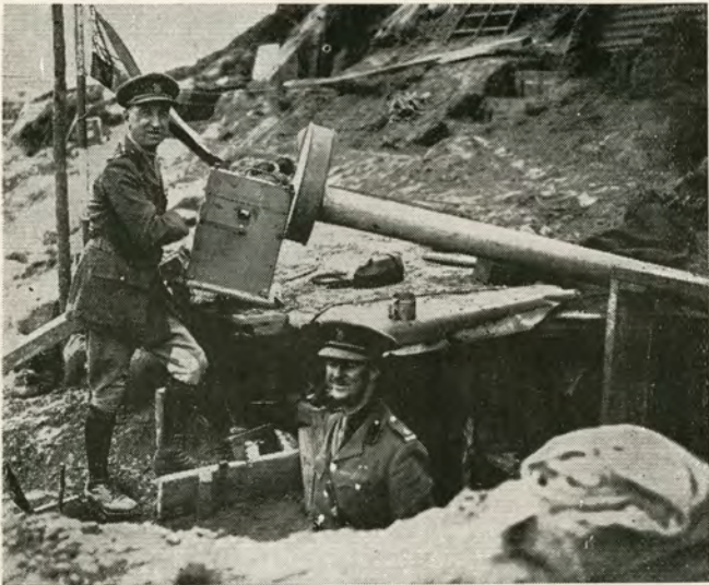
CAPTAIN "BILL" SHAUGHNESSY TESTING A GERMAN VENTILATING MACHINE. MAJOR WILLIS O'CONNOR IS SEEN JUST COMING UP FROM THE DUG-OUT.
