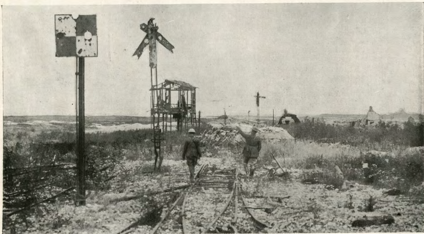
ALL THAT WAS LEFT OF A SMALL STATION NEAR LENS. THE PERMANENT WAY IS BADLY DAMAGED.
