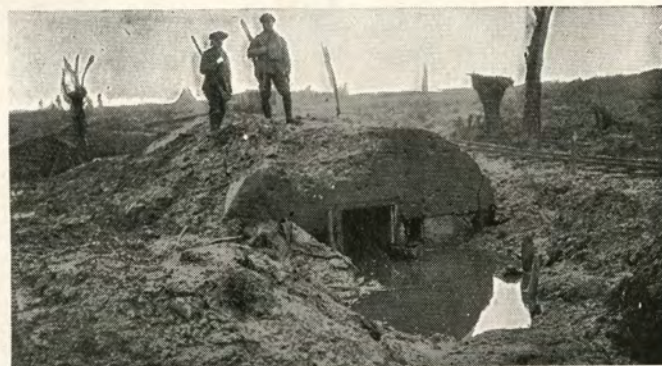
THESE CONCRETE STRONG-POSTS WERE USUALLY HALF SUNK LIKE THIS, AND THEREFORE PRESENTED A VERY SMALL TARGET.
