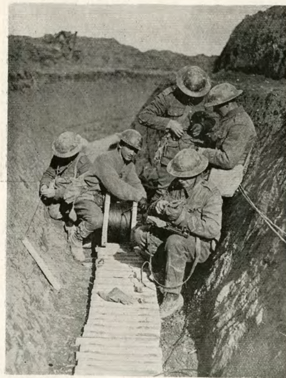
SIGNALERS REPAIRING WIRES IN A COMMUNICATION TRENCH NEAR THE FRONT LINE.
