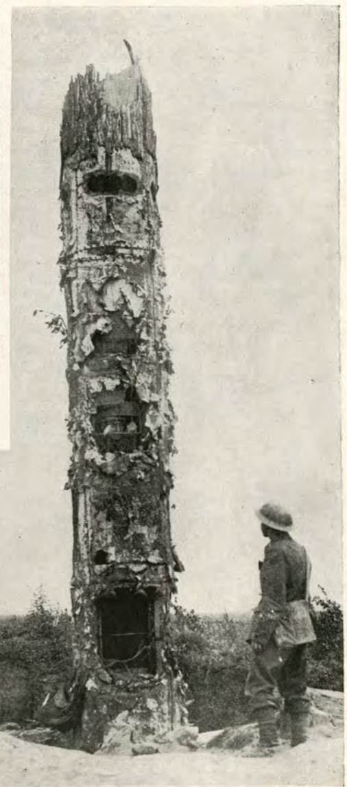
A GERMAN OBSERVATION POST MADE OUT OF A HOLLOW TREE. NOTE THE OFFICER INSIDE.
