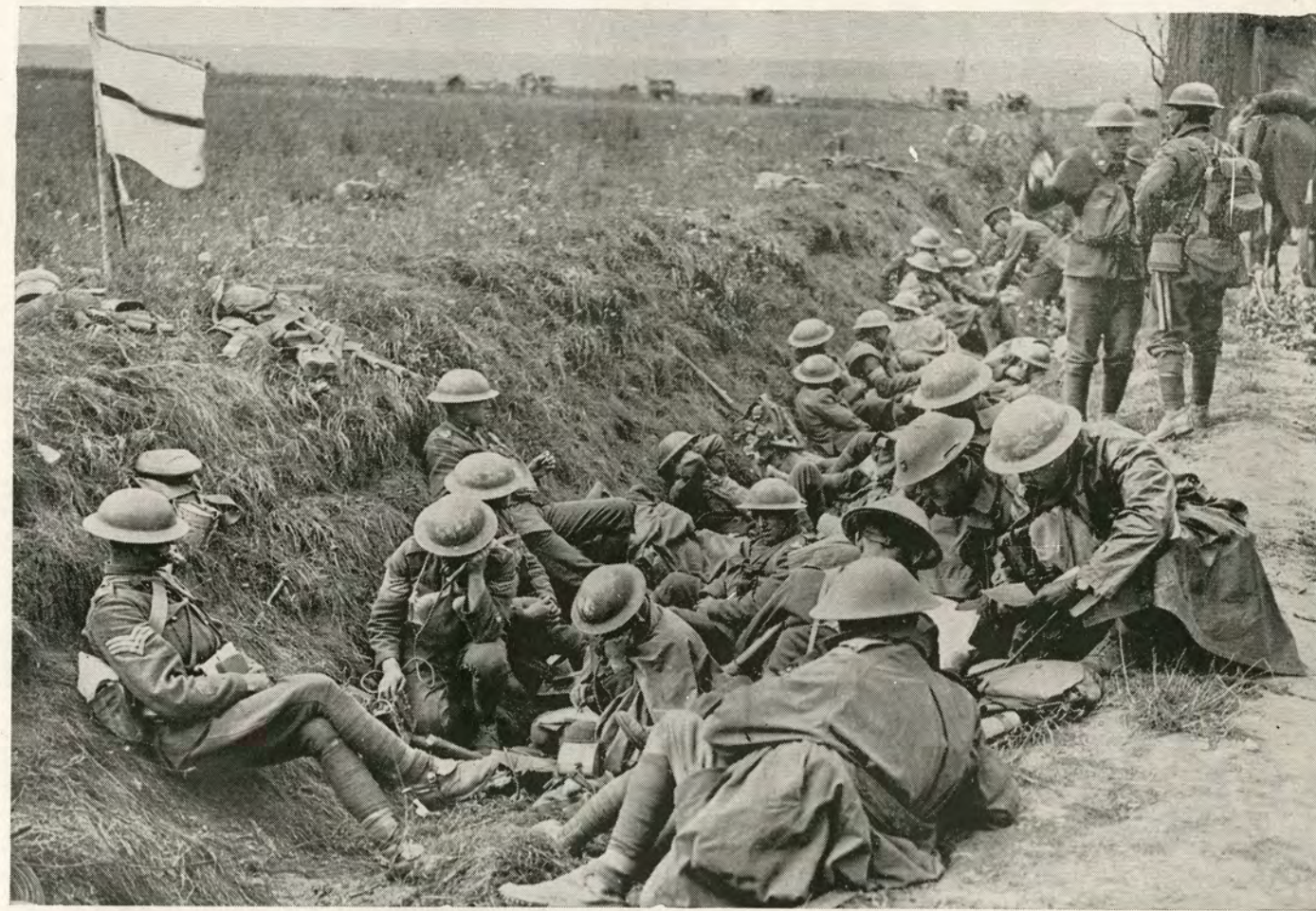
BRIGADE HEADQUARTERS DURING THE AMIENS ADVANCE.
