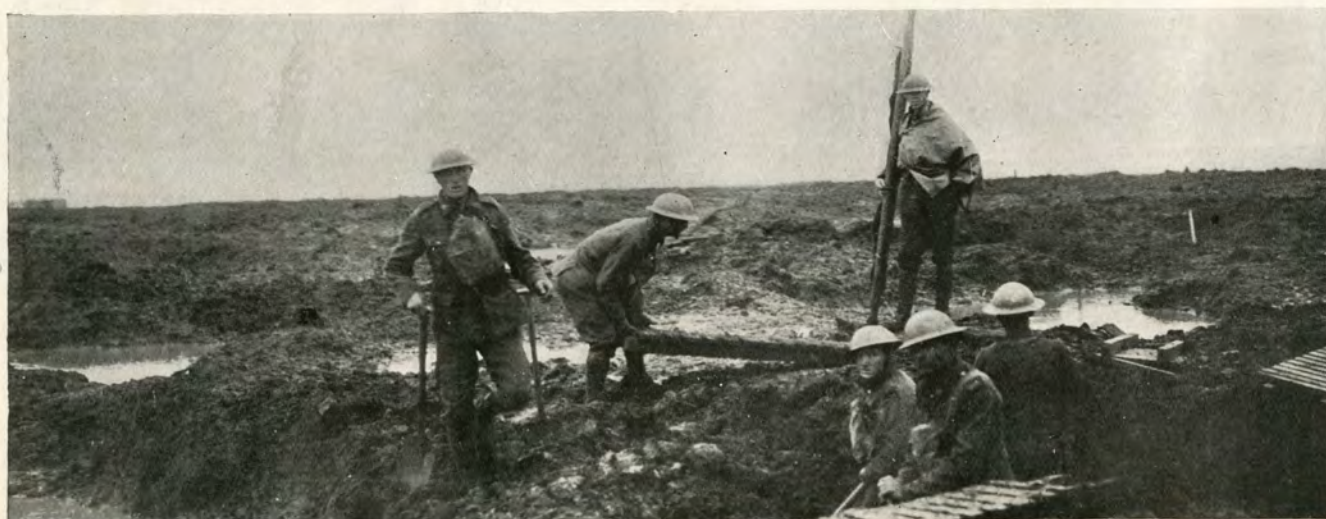
CANADIAN PIONEERS LAYING A TRACK OF DUCK-BOARDS AMONG THE MUD AND SHELL HOLES AT PASSCHENDALE OVER WHICH THE WALKING WOUNDED COULD COME OUT.
