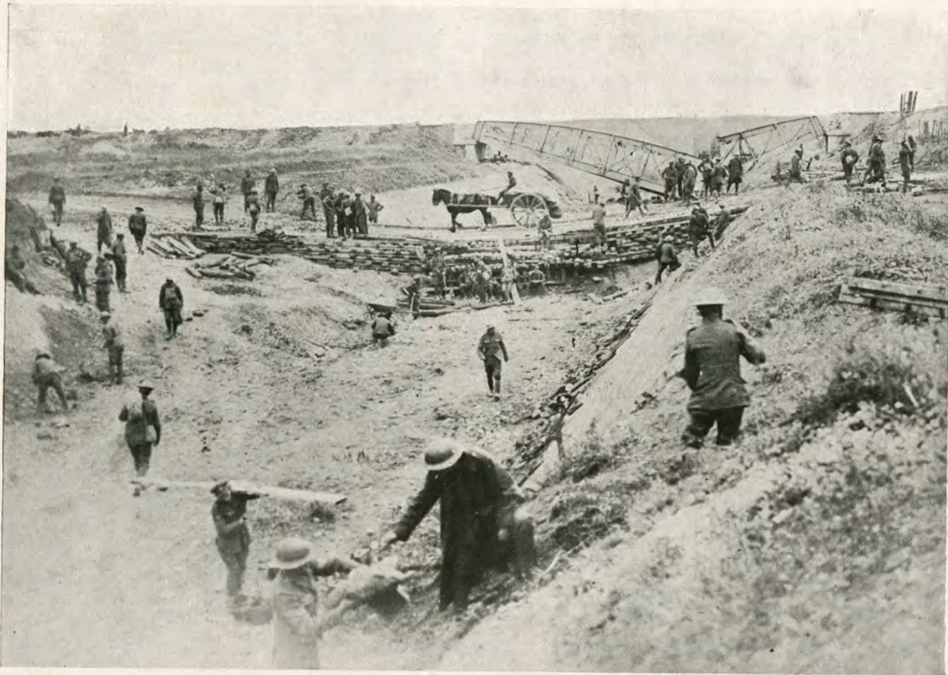
CANADIAN ENGINEERS CONSTRUCTING A BRIDGE ACROSS A RIVER ON THE ARRAS-CAMBRAI ROAD ON THEIR WAY TO CAMBRAI.
