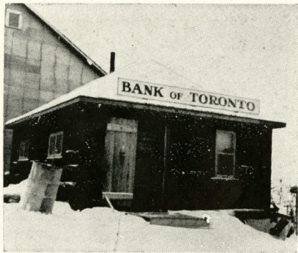
The spirit of pioneers is reflected in this picture of a log cabin branch of the Bank of Toronto, recently opened at Yellowknife, North West Territories. Some day the more luxurious banking accommodation we know will be available at this northern outpost of civilization.
