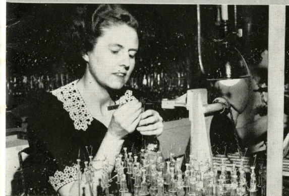
PROJECTION LAMPS FOR WAR The same lamp used in projection machines which flash your favourite movie star on the screen is in constant demand for war purposes. Cora Ashbough, left, of the Westinghouse Lamp Dept., is seen mounting filament coils for the 500-watt projection lamp supplied to the R.C.N.V.R., the Army and the R.C.A.F. Right, movies used for training purposes.
