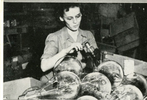
FLOODLIGHTS GUIDE PLANES Big lamps for a big job. Soldering base leads to these 1000-watt Westinghouse floodlights is Erla McGraw, left, whose efforts are motivated by the fact that she's doing important war work. The lamps are used almost exclusively for floodlighting docks, railroad loading areas and hundreds of airports like the one shown on the right.
