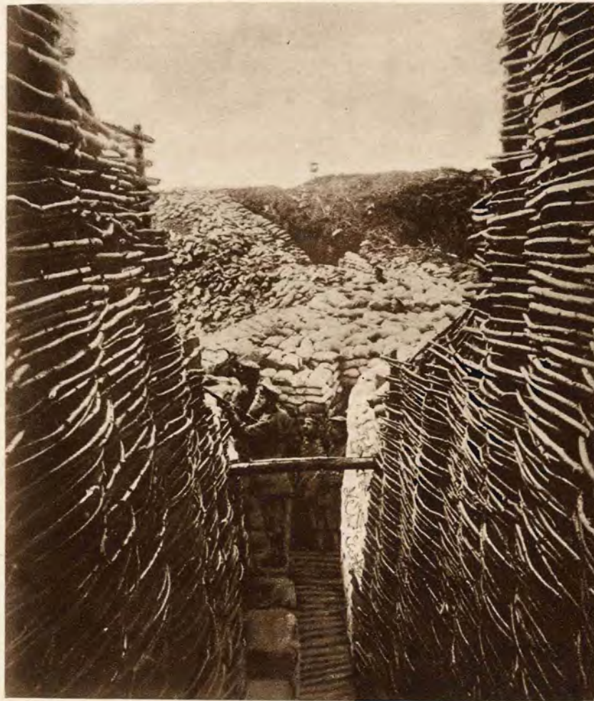
DUG DEEP; WITH WILLOW WITHE WALLS: A GERMAN TRENCH IN FLANDERS.
