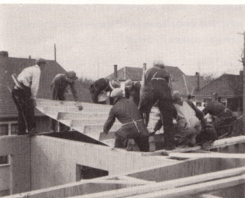
Ceiling sections built in large panels.
