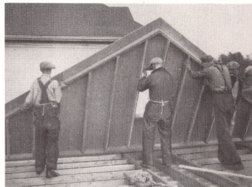
Gable end in one piece—slides into place.
